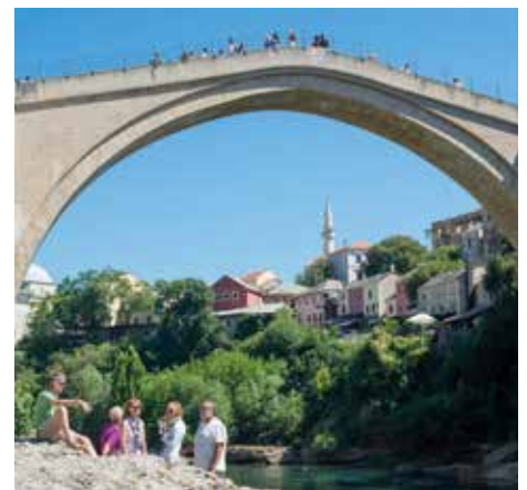
MOSTAR BRIDGE, BOSNIA & HERZEGOVINA
