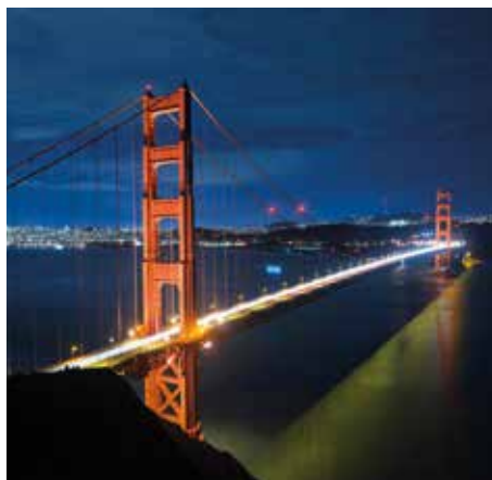
GOLDEN GATE BRIDGE
