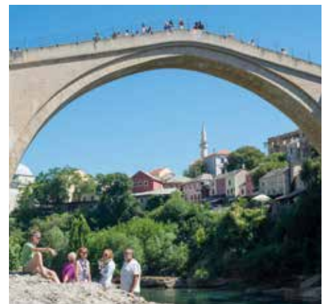
MOSTAR BRIDGE, BOSNIA & HERZEGOVINA
