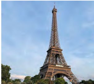
@CHANTAL_INSIGHT EIFFEL TOWER, FRANCE
